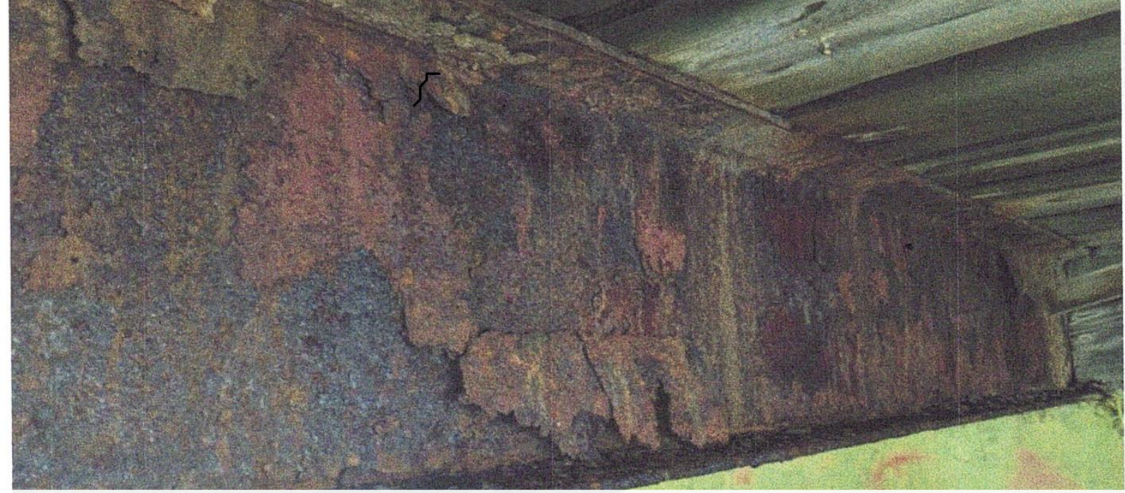
Corrosion Typical of all Beams
